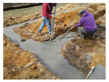
However, some excavators, not being Licensed General Contractors, unfortunately make the vertical leg of such step-downs too close to the surface of the ground. This can result in frost heave during harsh mountain winters, cracking the foundation, fracturing the foundation wall, as well as transferring other movement problems throughout that portion of your structure, including breaking
