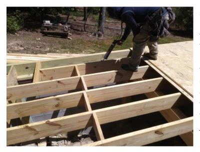
sized your floor joists, it is unlikely that you will ever hear or feel floor squeaks or nail pops. Your subfloor sheathing becomes bonded to your floor joists, turning them into a sort of double tee, system like precast concrete systems. In other words, your floor sheathing works together with your floor joists to form a stiffer floor that hardly has any detectable bounce in it when you walk across it.
